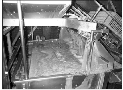
Crates moving into main wash booth; water recycling via a run down screen and make up tank
