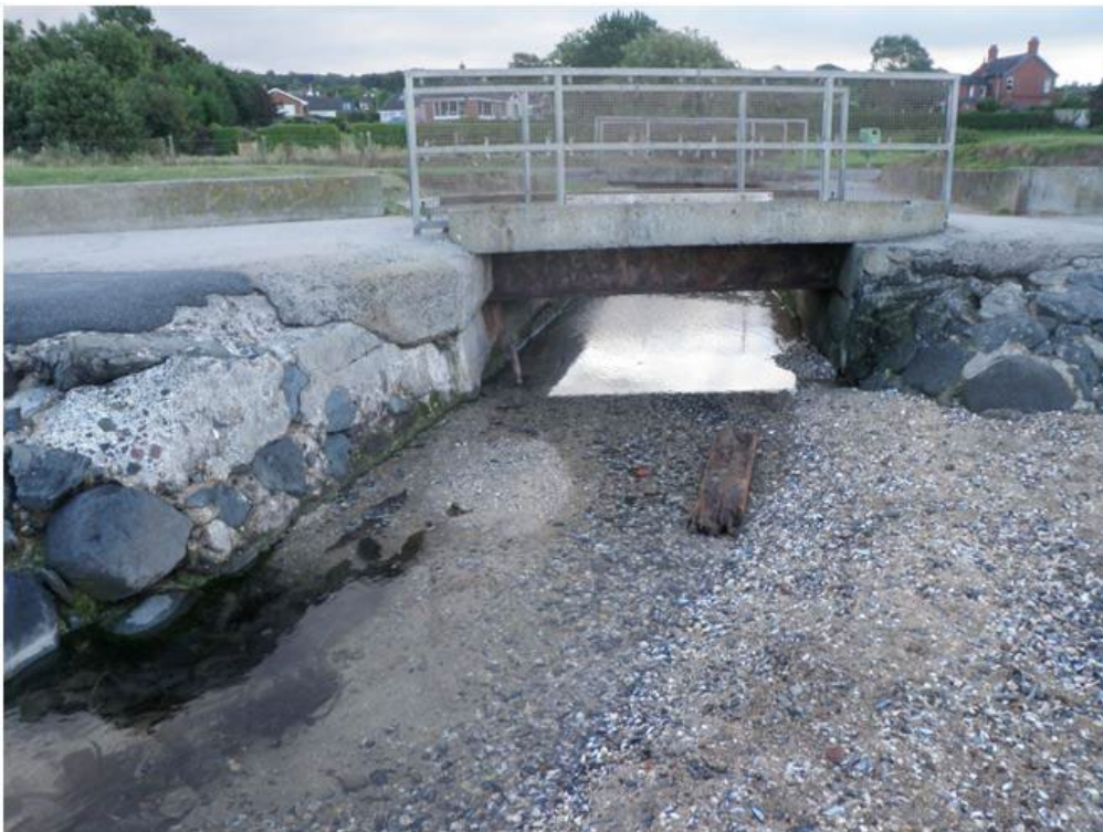
Figure 32. Culverted watercourse. Site of freshwater sample BLS FW06.
