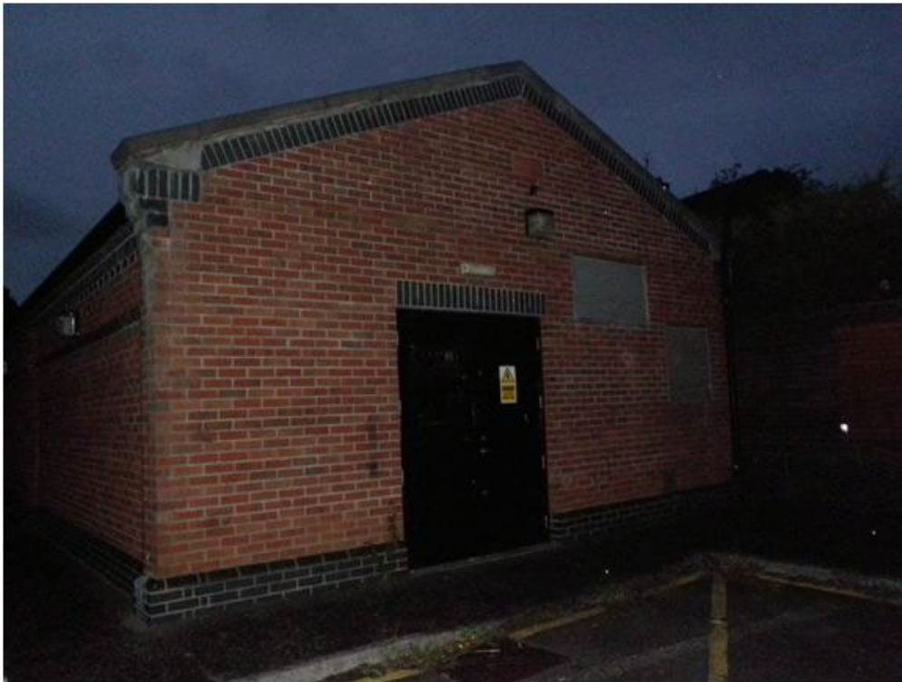
Figure 42. Presumed sewage pumping station in Helen's Bay Beach car park.
