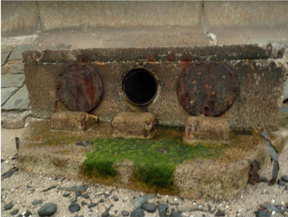
Figure 23. Three openings in concrete structure, two blocked up. No flow.
