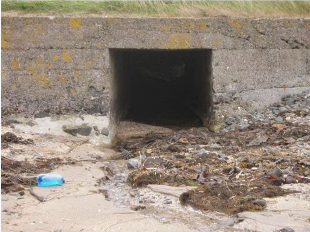
Figure 37. Culverted watercourse. Site of freshwater sample BLS FW09.
