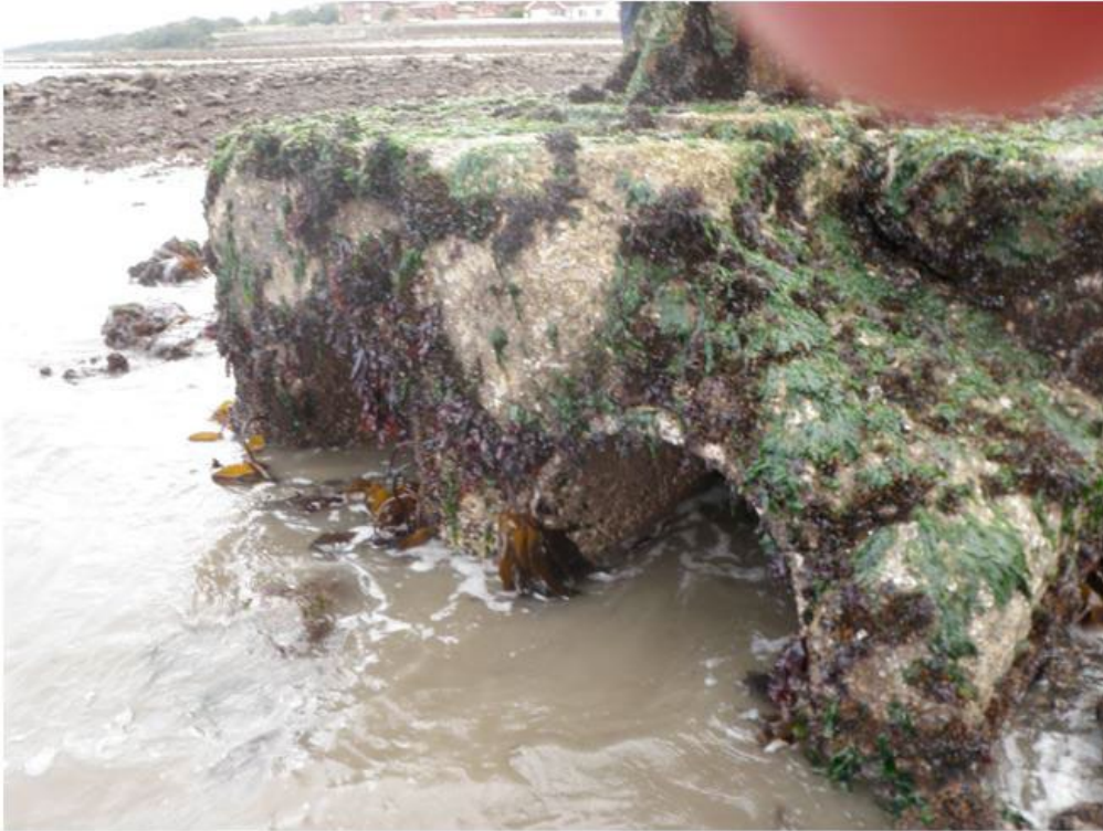
Figure 35. Ends of two pipes. Site of seawater sample BLS SW02.
