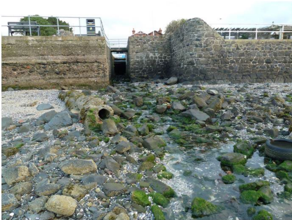
Figure 6. Outfall pipe and watercourse. Site of freshwater sample BLNS5.
