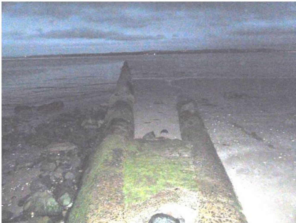
Figure 18. Long and short outfall pipes with no evidence of flow. Seawater sample BLNS20 taken at end of long pipe.
