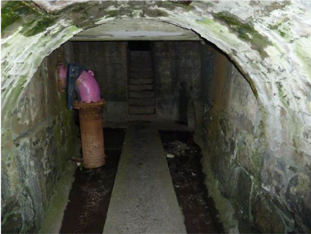
Figure 19. Two watercourses in culvert under railway line. Site of freshwater sample BLNS18.
