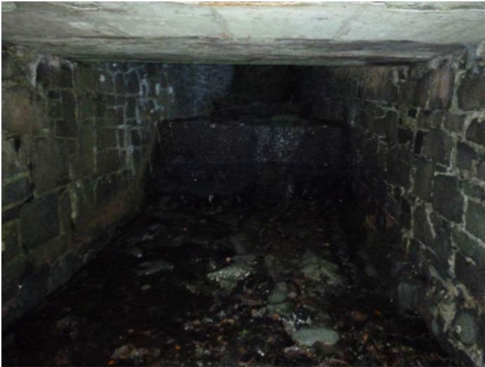
Figure 3. Small watercourse running through channel in sea defences. Site of freshwater sample BLNS1.
