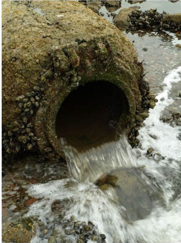
Figure 27. Outfall from Green Island STW.
