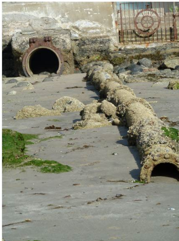
Figure 14. Two pipes, neither with flow at time of survey.
