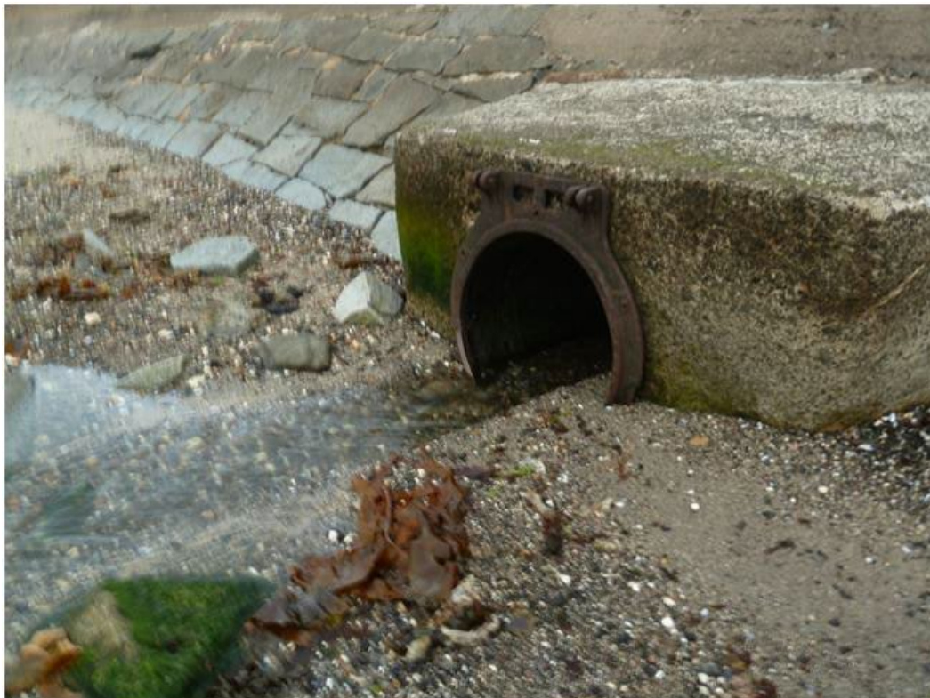
Figure 24. Culverted watercourse. Site of freshwater sample BLNS23.
