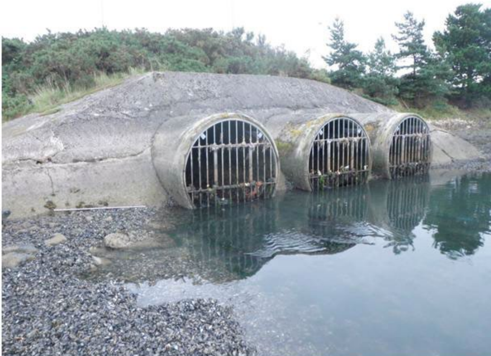
Figure 46. One of two sets of three outlets from lagoon.
