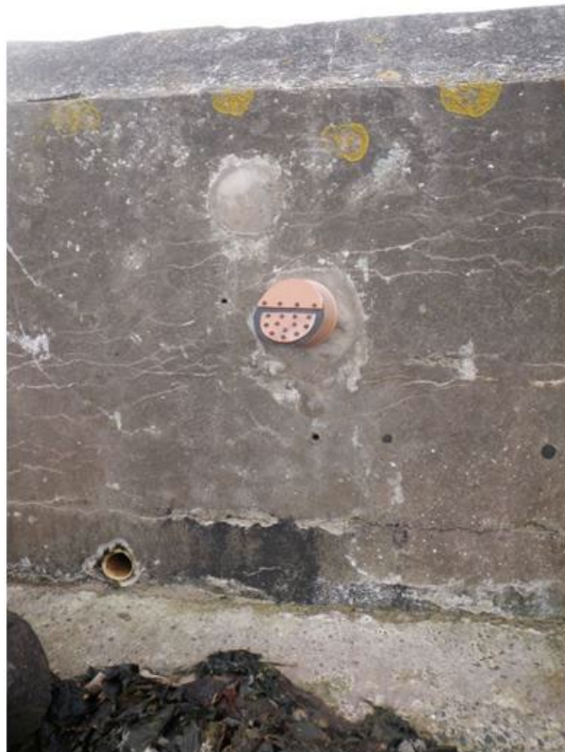
Figure 36. Flap valve in sea wall.
