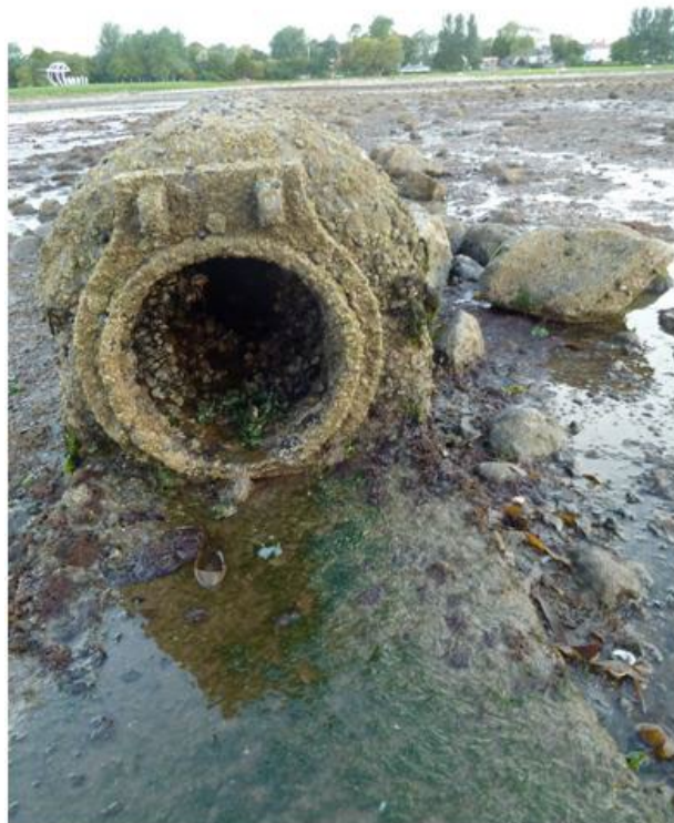
Figure 10. End of long outfall pipe. Site of freshwater sample BLNS10.
