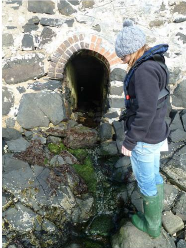
Figure 15. Culverted watercourse. Site of freshwater sample BLNS15.
