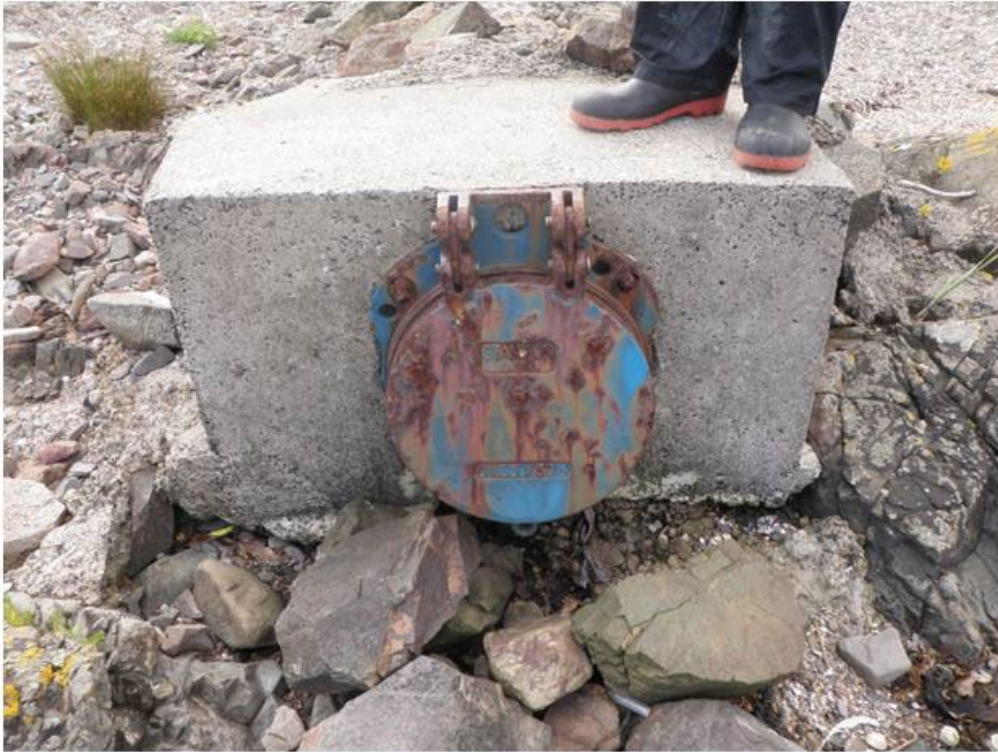
Figure 39. Flap valve on end of pipe. No flow at time of survey.
