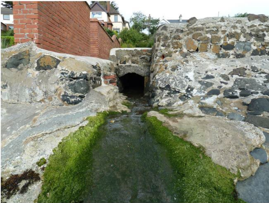
Figure 16. Culverted watercourse. Site of freshwater sample BLNS16.
