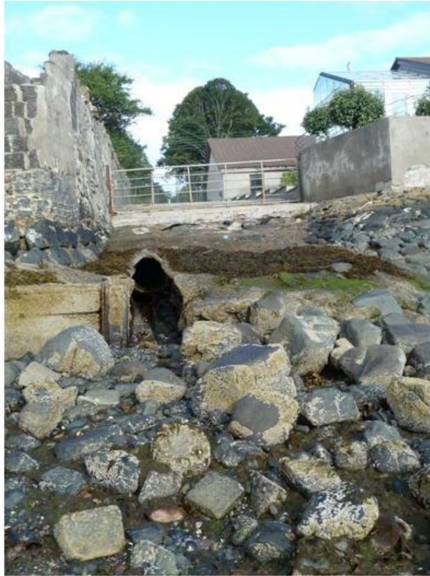
Figure 13. Culvert under road. Site of freshwater sample BLNS13.
