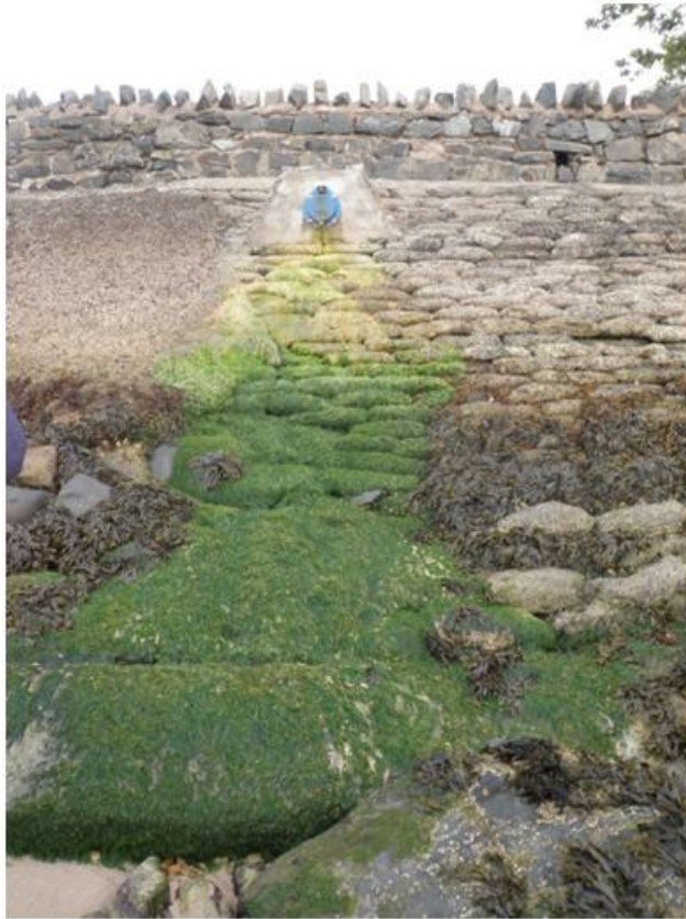
Figure 33. Flap valve with signs of recent flow.
