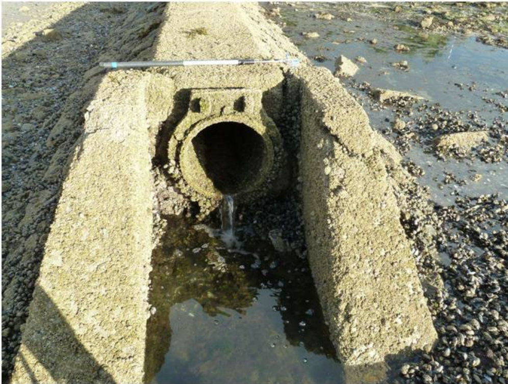
Figure 9. Outfall pipe. Site of freshwater sample BLNS9 and mussel sample BLNSM2.
