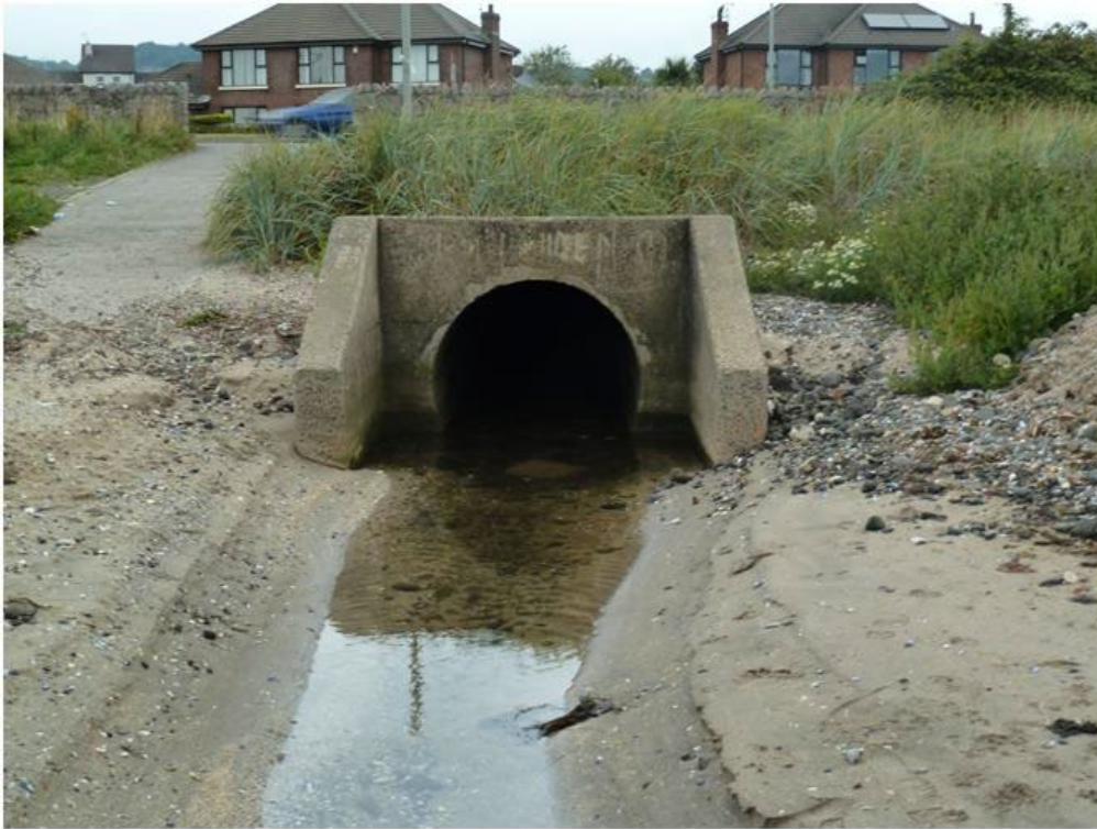
Figure 25. Culverted watercourse. Site of freshwater sample BLNS24.
