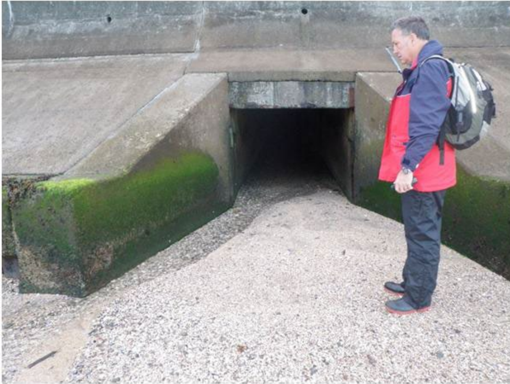
Figure 29. Culverted watercourse. Site of freshwater sample BLS FW03.
