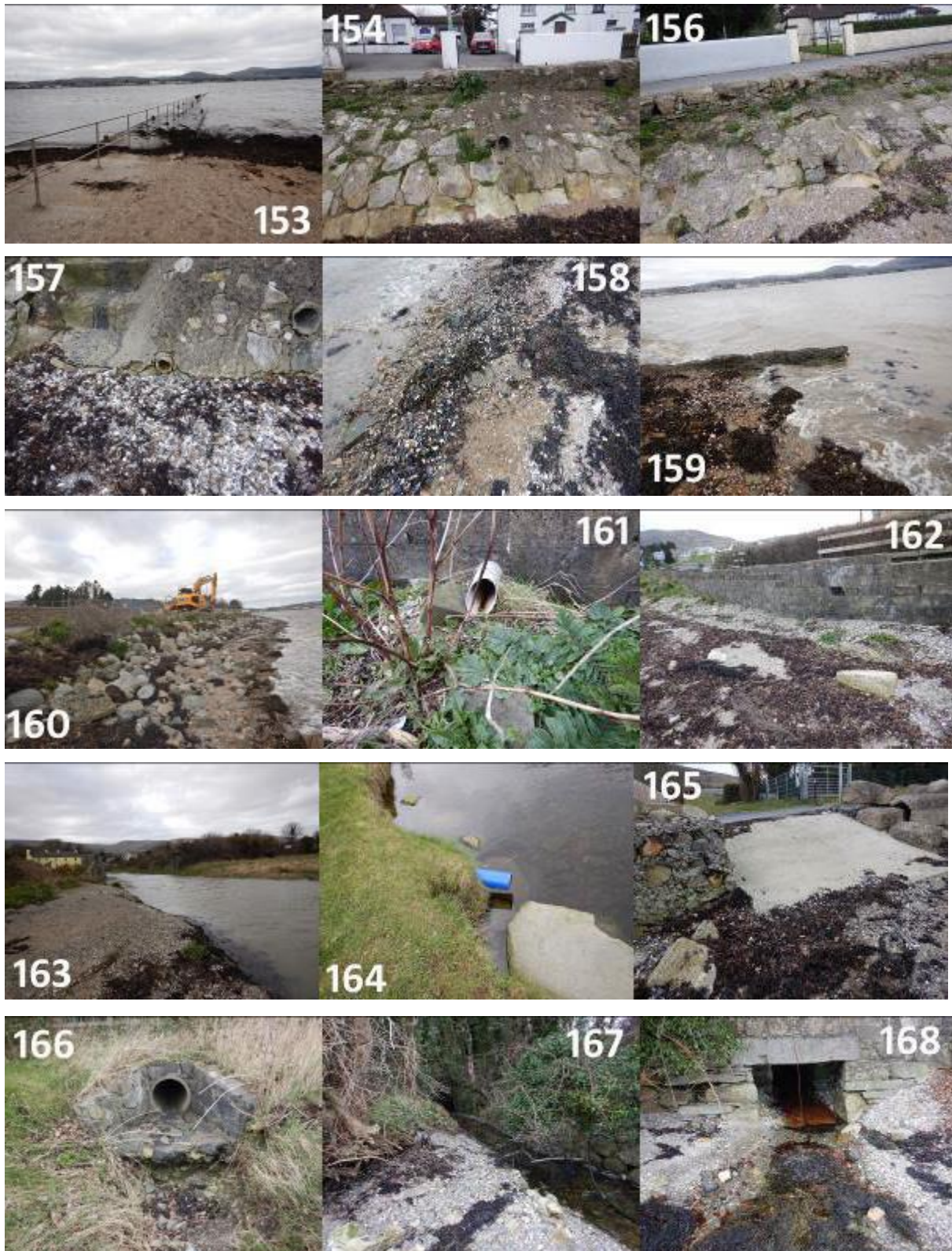
Figure 4.63: Images of features identified in shoreline survey 153-168, no image for feature 155 (numbering refers to Table 4.8).
