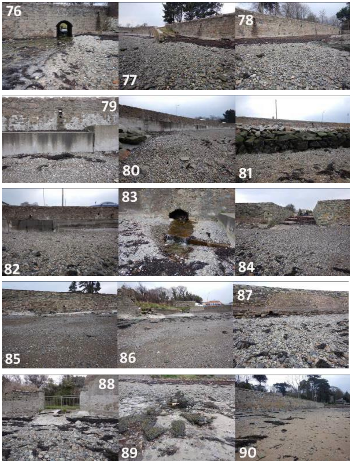
Figure 4.113: Images of features identified in shoreline survey 113-113
