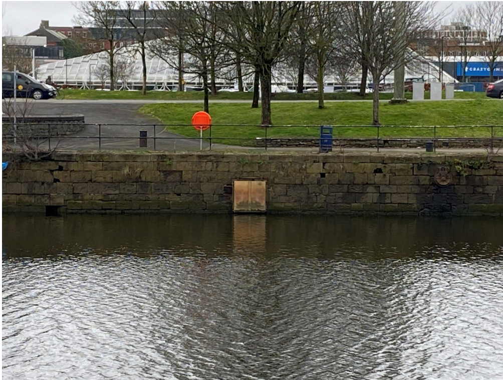
Figure 17 Parc Tawe outfall confirmed. No flow observed during survey.
