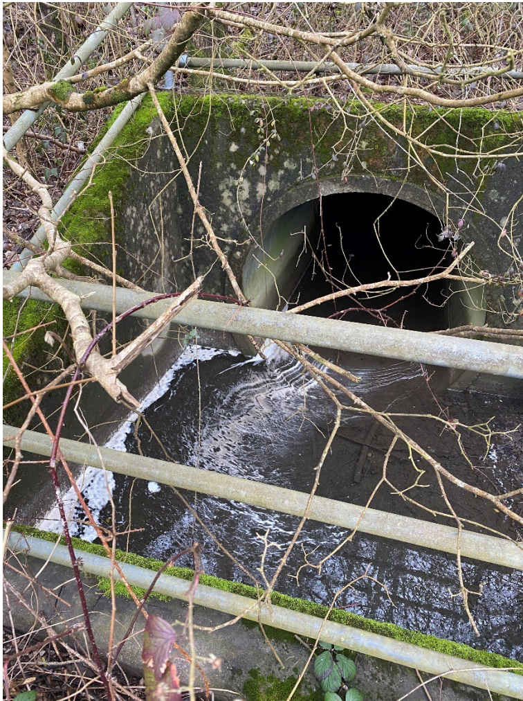
Figure 21 Surface road drainage identified during the shoreline survey path route up the River Tawe. Observed to be flowing on the day of survey with a strong smell and surface foam.
