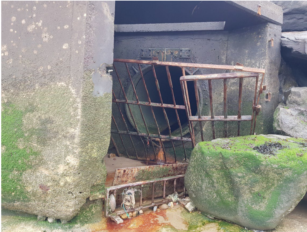
Figure 13 Outfall 2 seaward. Identified during shoreline survey. Flow observed on survey day. Anthropogenic material in surrounding area and water staining visible from flow of water. Location of water sample SCPH23013.
